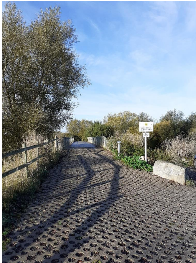
5. Huish Bridge facing west south west, between points A1 and A2
