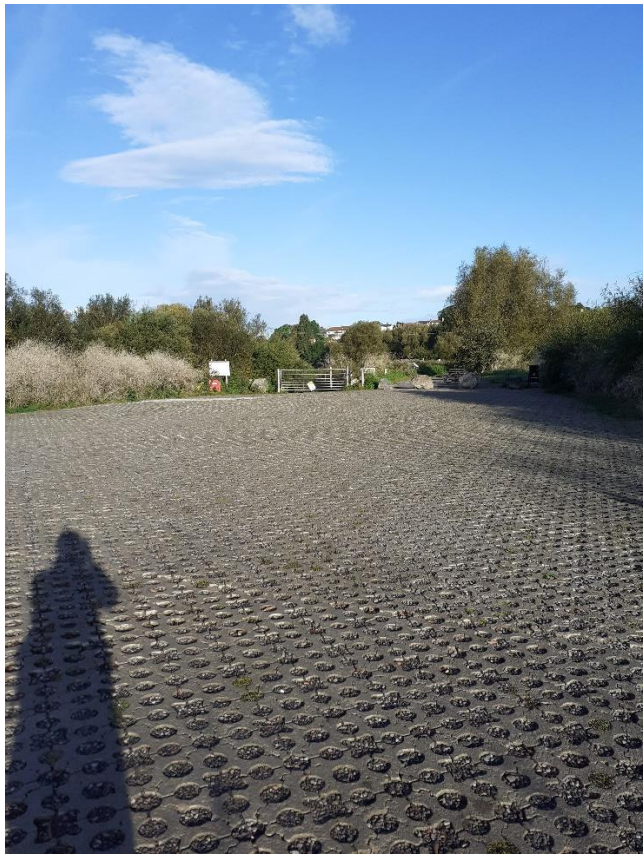
4. Car park at Huish Bridge, between points A1 and A2
