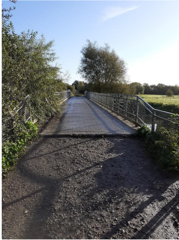
7. Huish Bridge facing east north east, between points A1 and A2
